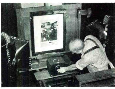
Photographic engineer using a Totalux to integrate light intensity with time, in reference to exposure in photography.
