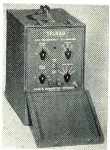
Special models designed for use under adverse conditions are available equipped with two precision crystals that have been ground to produce exact frequencies of 100 and 1,000 kc. and tested for efficient operation at temperatures from—35° to 55° Centigrade and have temperature co-efficients of maximum drift of only 2 and 3 cycles per megacycle per degree Centigrade respectively.
